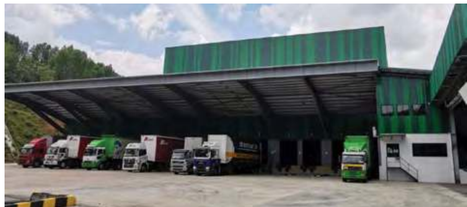
A building with small environmental footprint while providing occupants a healthy & comfortable indoor and outdoor environment. The roof overhang in front of building acts as effective shading device to internal area blocking direct sunlight, further reduce the heat gain in the internal building.
