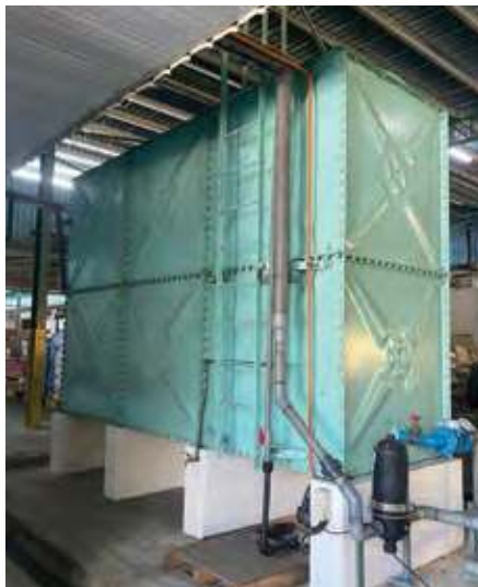
RAINWATER HARVESTING SYSTEM AT TAIPING PLANT
